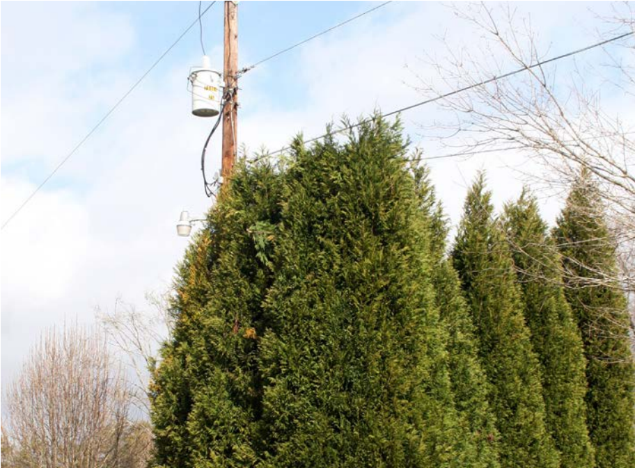
Pruning under lines
