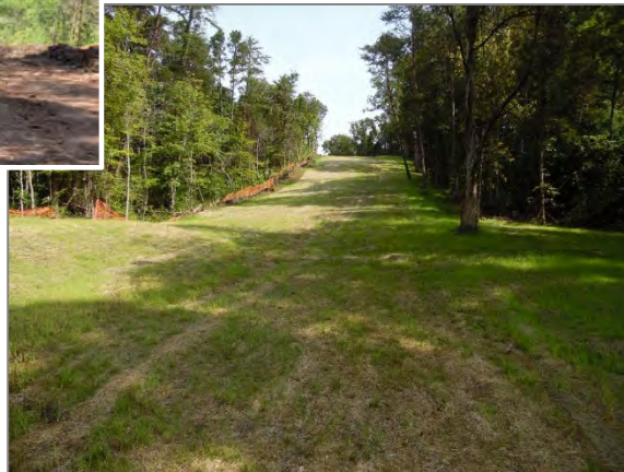
Main Installation Completed August 2018
