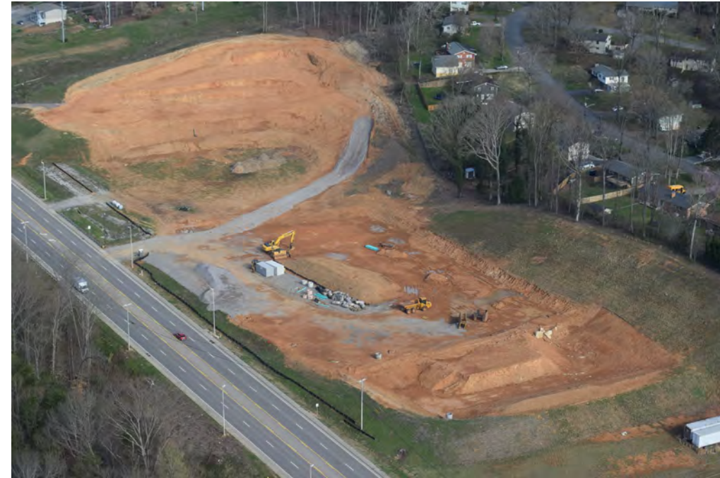
Western Ave. Substation Site Development – March 23
