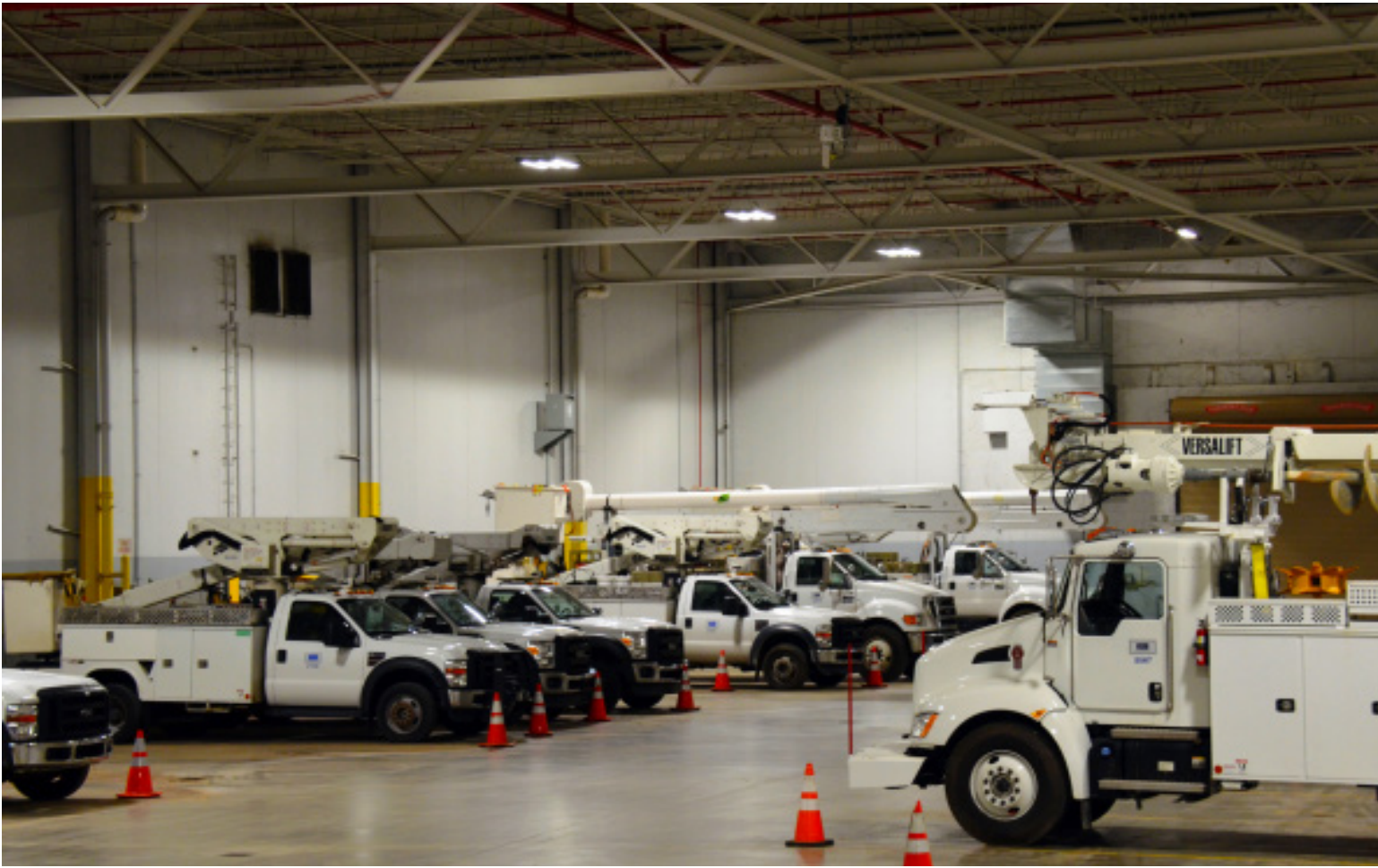
Above: In the Overhead Construction truck bays, more than 50 metal halide high-intensity discharge (HID) light fixtures have been replaced with light-emitting diode (LED) fixtures controlled by occupancy sensors.
