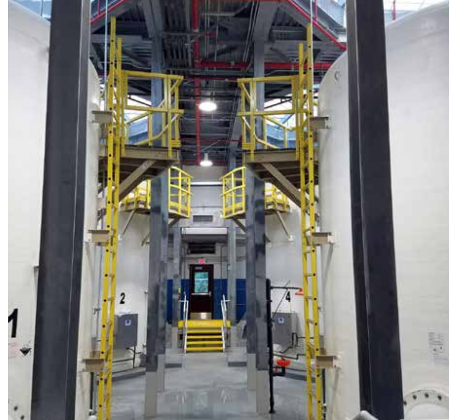
Four hypochlorite tanks and multiple feed pumps help ensure continuous water treatment even if there is an equipment failure.
