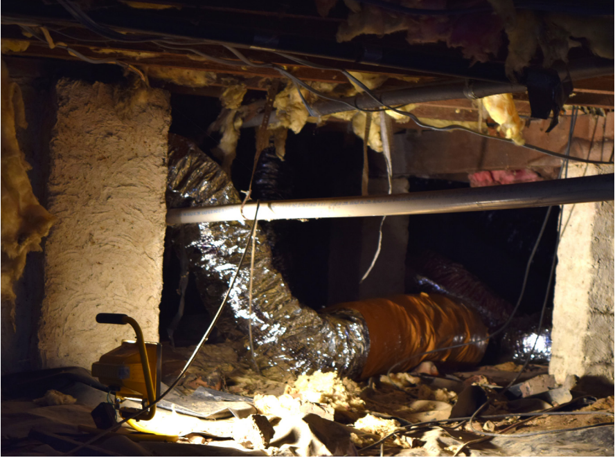
Above: Through KUB's low-income weatherization programs, problems like damaged ductwork and insulation are remedied, making homes more efficient and lowering energy bills.
