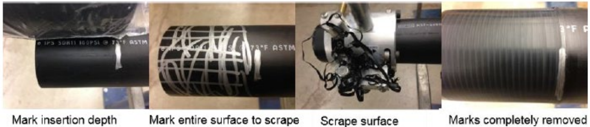
Figure 6. Correct Scraping
