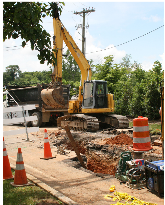
Pictured above is a Century II infrastructure improvement project that involved natural gas, water, and wastewater pipeline upgrades along 1.5 miles of Lyons View Pike.
