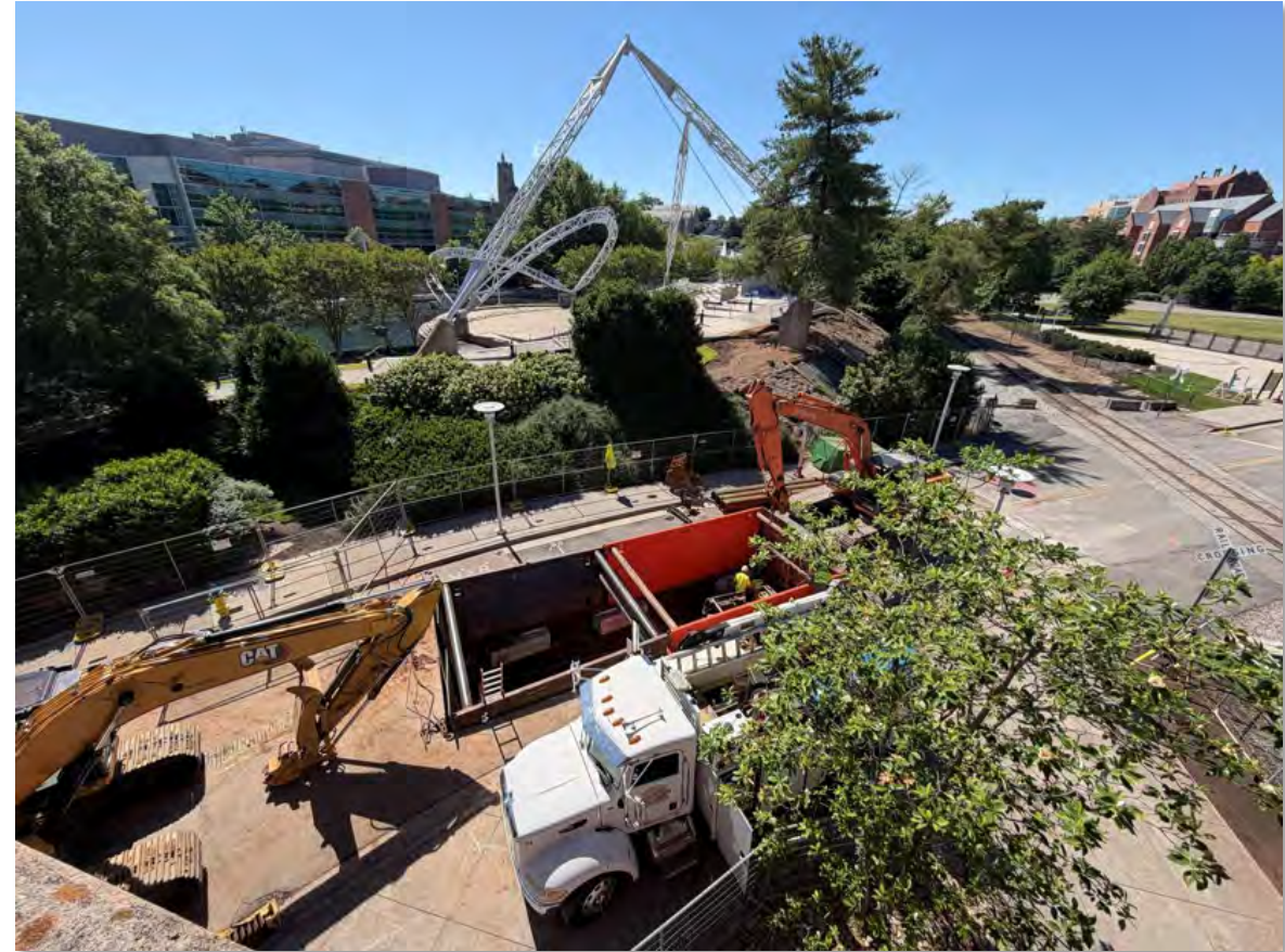
Casing installation at World's Fair Park
