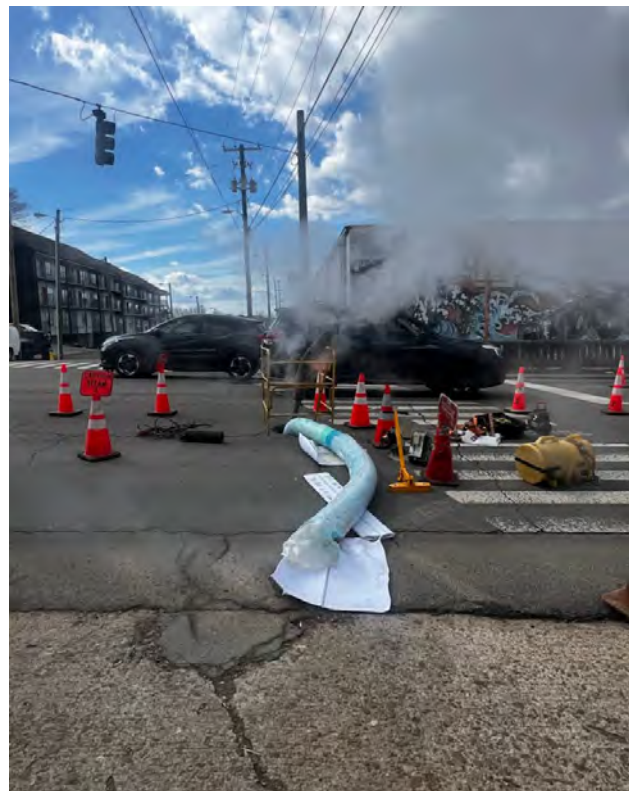
Fort Sanders Sewer Replacement Phase 1
