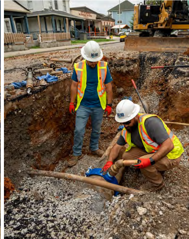
Fort Sanders Water Main Replacement Project Phases 1 & 2
