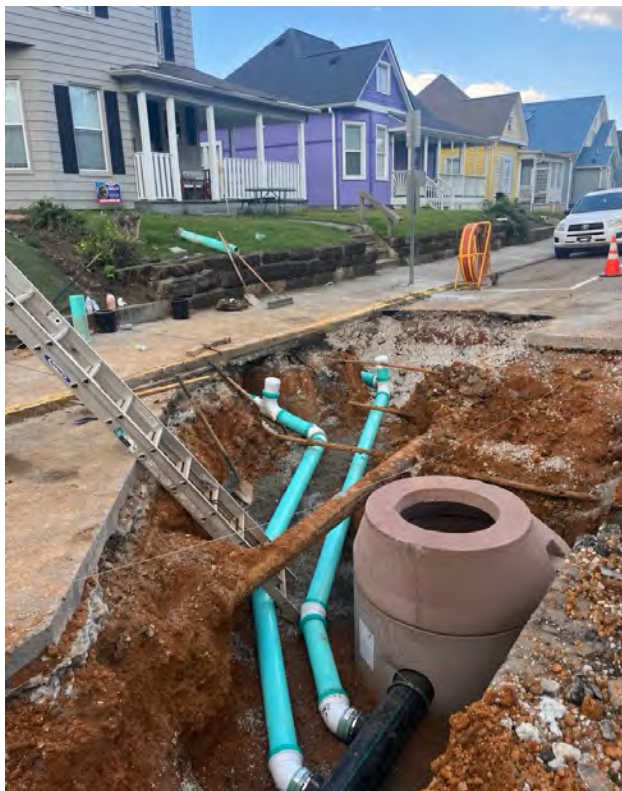
Fort Sanders Sewer Replacement Phase 2
