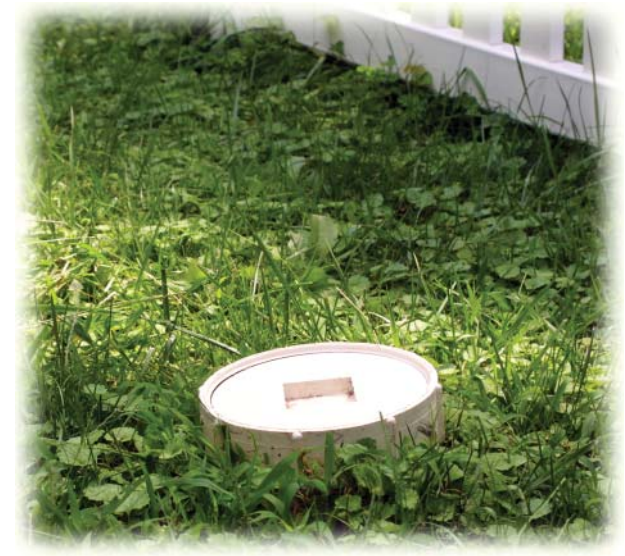
Properly maintained sewer lateral cleanout caps keep out debris that can lead to blockages.
