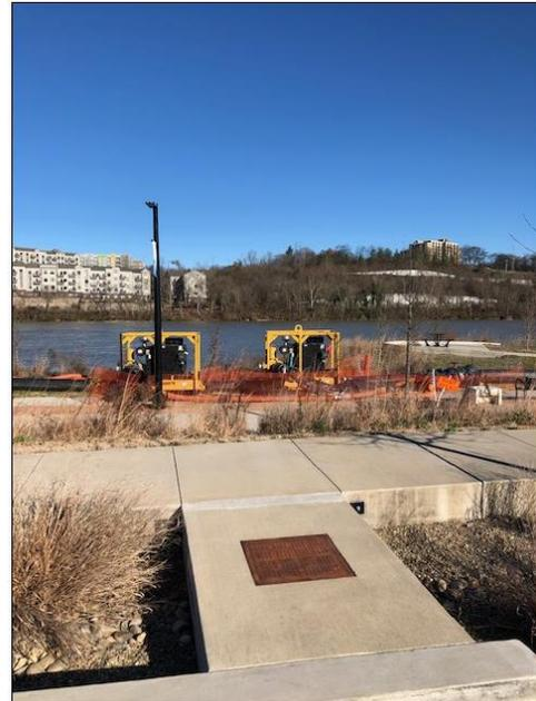
***Above-ground bypass piping with cross-over ramp (left) and pumping equipment (right) set up in Suttree Landing Park last winter as part of a wastewater rehabilitation project.***
